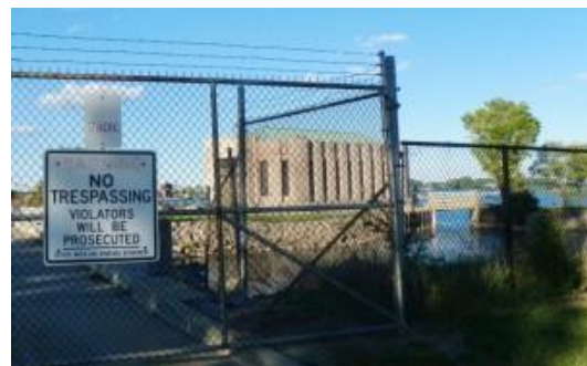
DWSD facility on Belle Isle.
