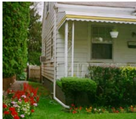
Downspout Disconnection
