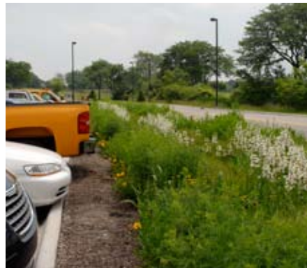
Parking Lot Bioswale
