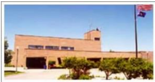
Thumb Correctional Facility mainly Houses younger prisoners at Level 2
